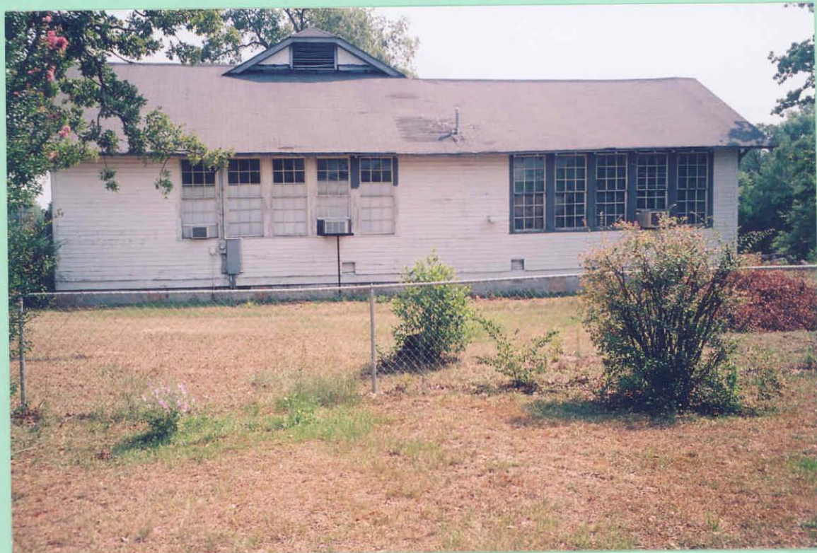
West View of Classroom #3 & Lunchroom
