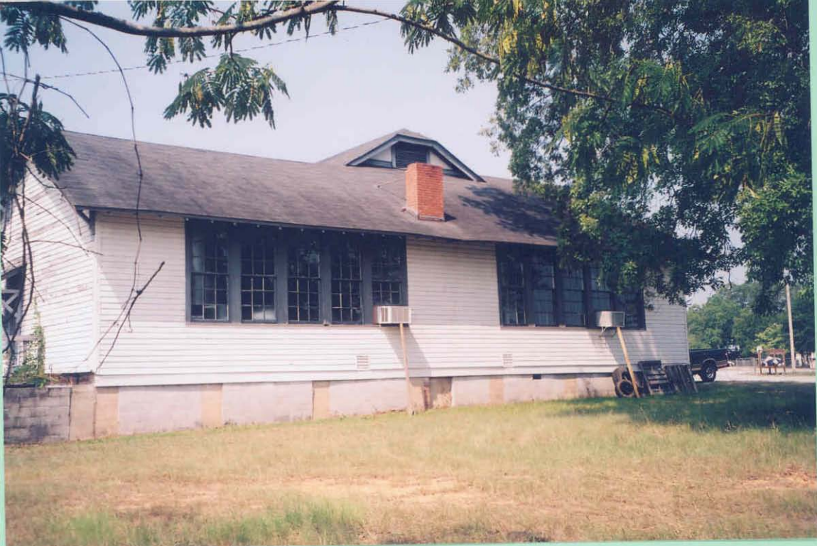
East View of Classrooms # 1 & #2
