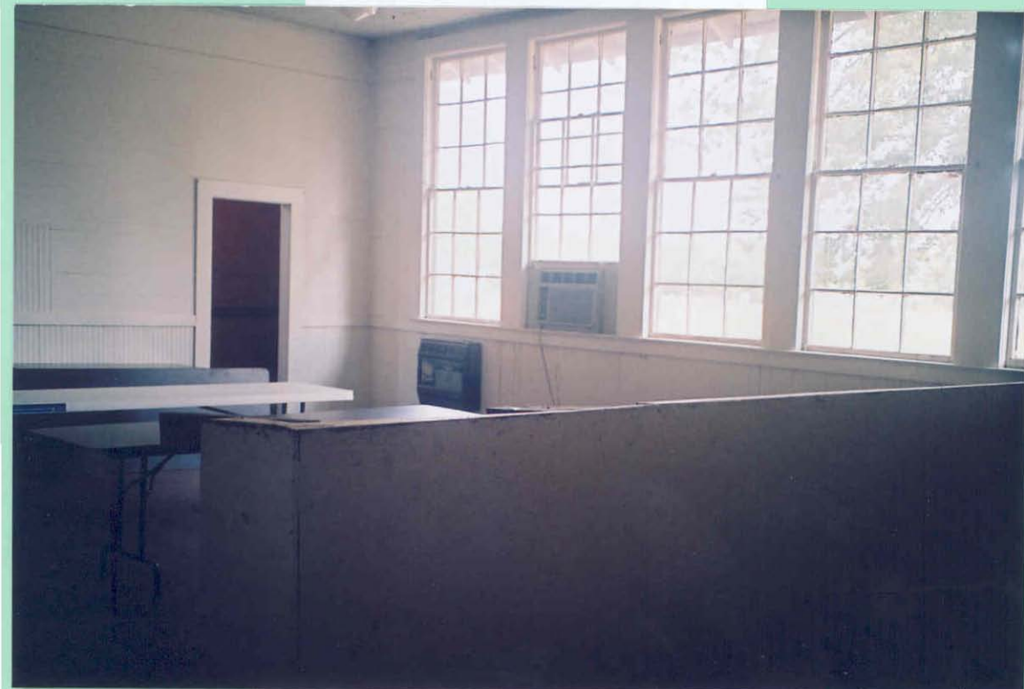
Original Cloakroom Five Banks of Original Tall Windows Original Beadboard Walls & Pine Floors Original Blackboards & Six-Panel Wood Doors
