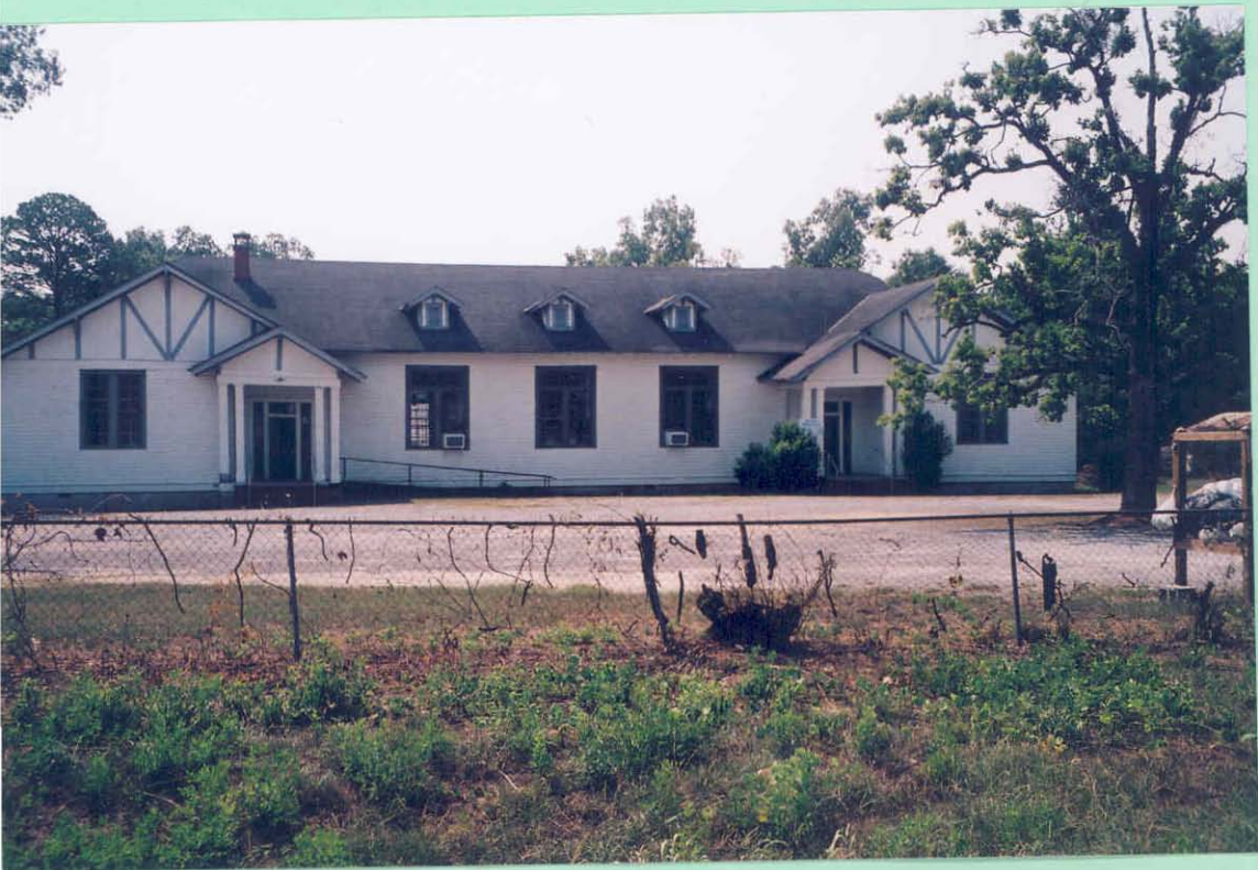
Front North View
