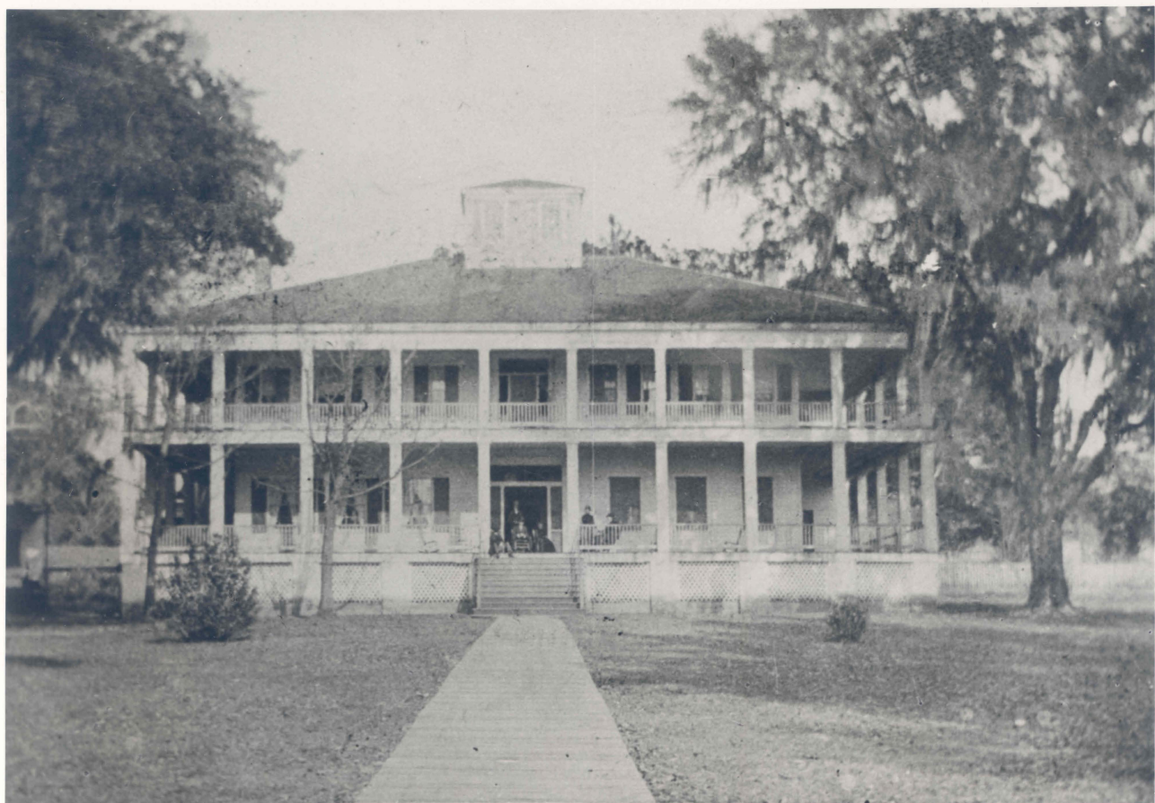
Date of Photograph - approximately 1900-1905 - Front elev.
