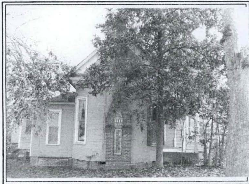
PHOTO NO. 5B : WEST ELEVATION SHOWING EXTERIOR DETAILS.
