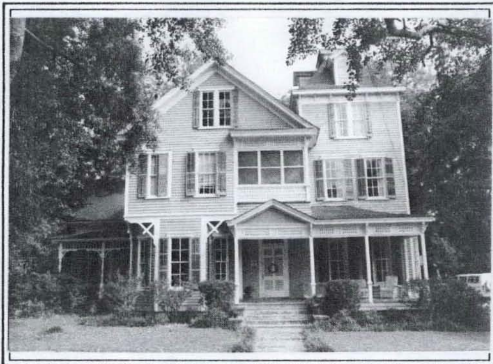
PHOTO NO. 1 : FRONT ELEVATION SHOWING VICTORIAN DETAILS AND ENVIRONMENTAL SURROUNDINGS.
