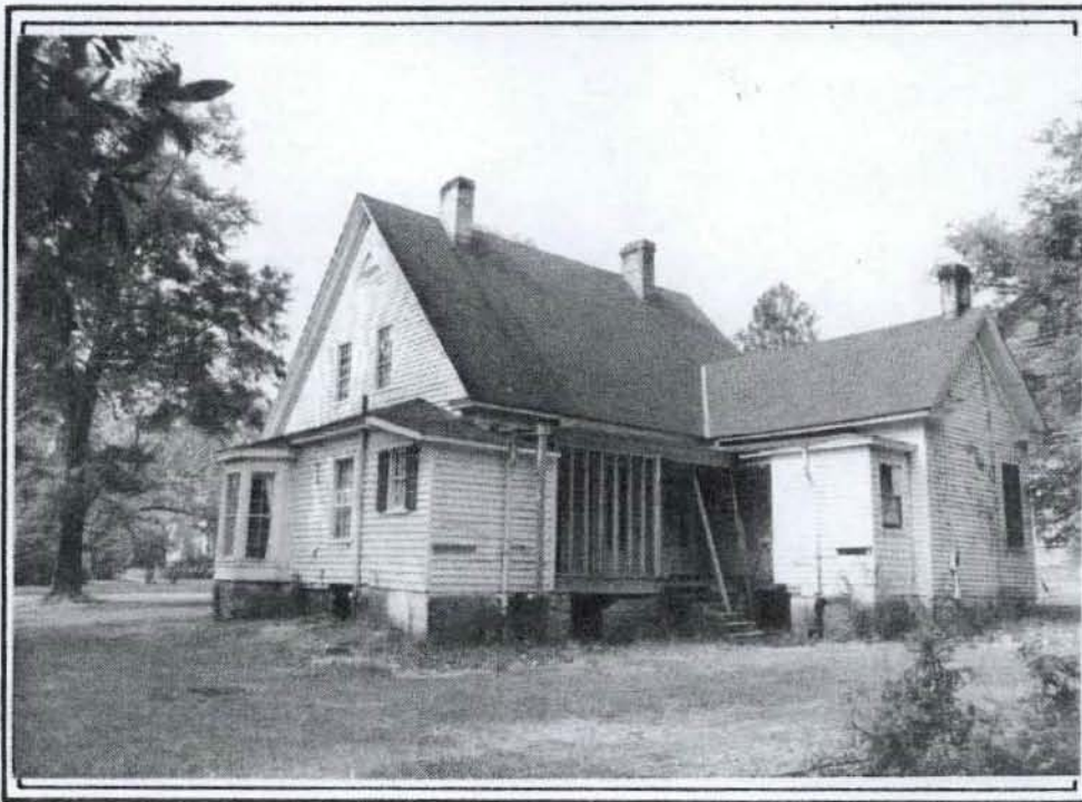
PHOTO NO. 4 : REAR ELEVATION SHOWING EXTERIOR ALTERATIONS.
