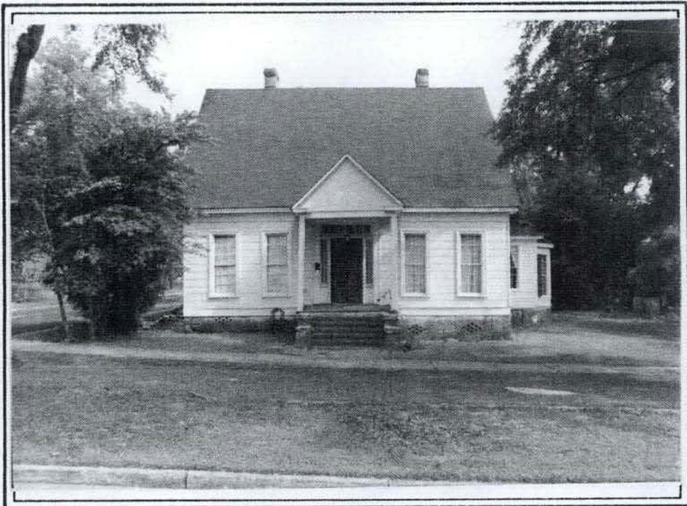
PHOTO NO. 1 : FRONT ELEVATION SHOWING EXTERIOR DETAIL AND THE ENVIRONMENTAL SURROUNDINGS.
