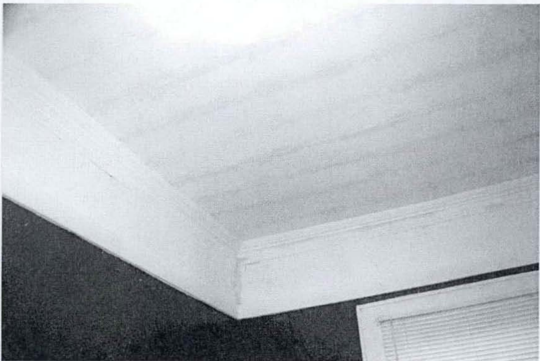
6. Interior, 1st floor parlor, camera facing northeast 7. Photo #12
