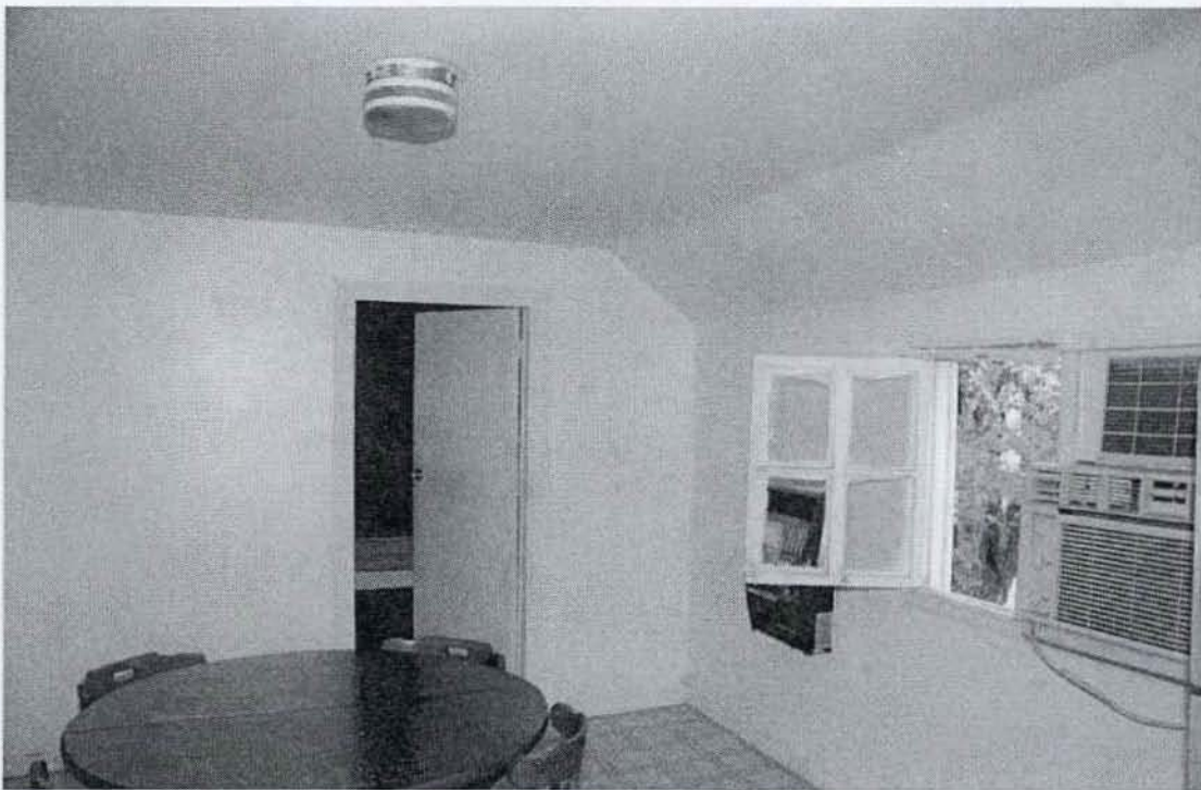
6. Interior, 2 nd floor, rear wing, camera facing northwest 7. Photo #16
