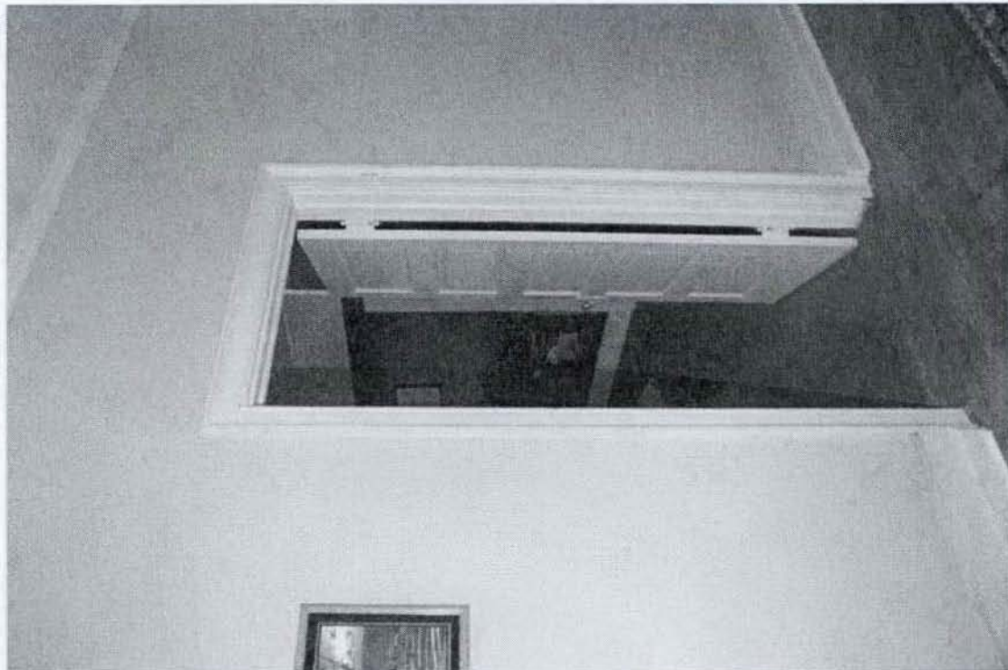
6. Interior, 1st floor hallway, camera facing southwest 7. Photo #09
