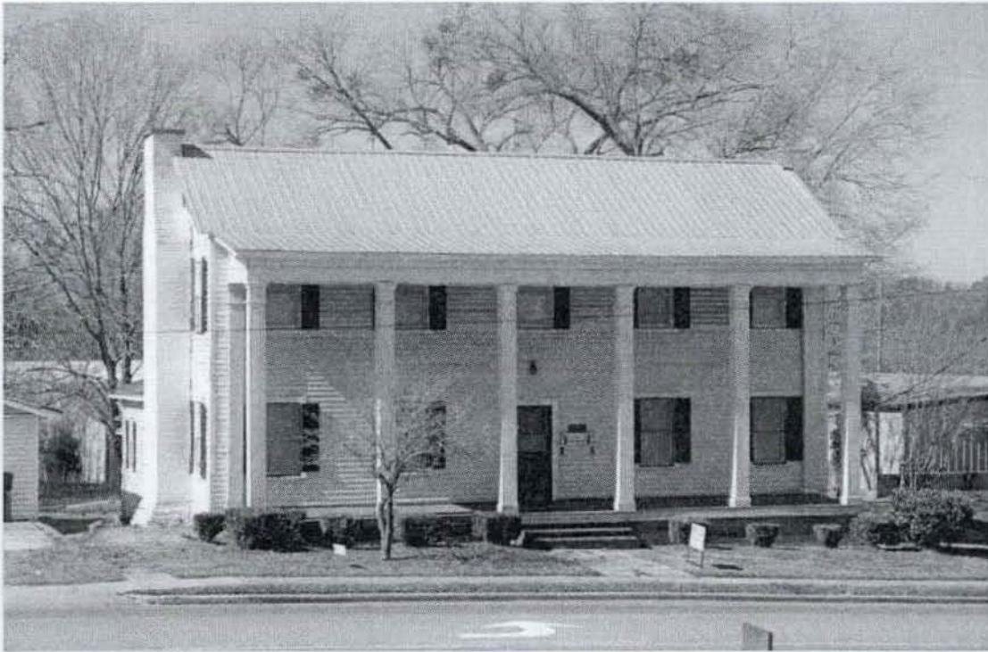
6. Exterior, East façade, camera facing west 7. Photo #01
