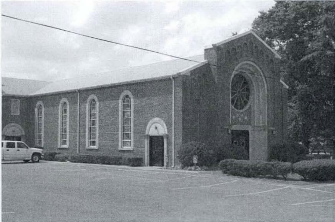
6. Exterior, east façade (right) and south elevation, camera facing northeast 7. Photo #01
