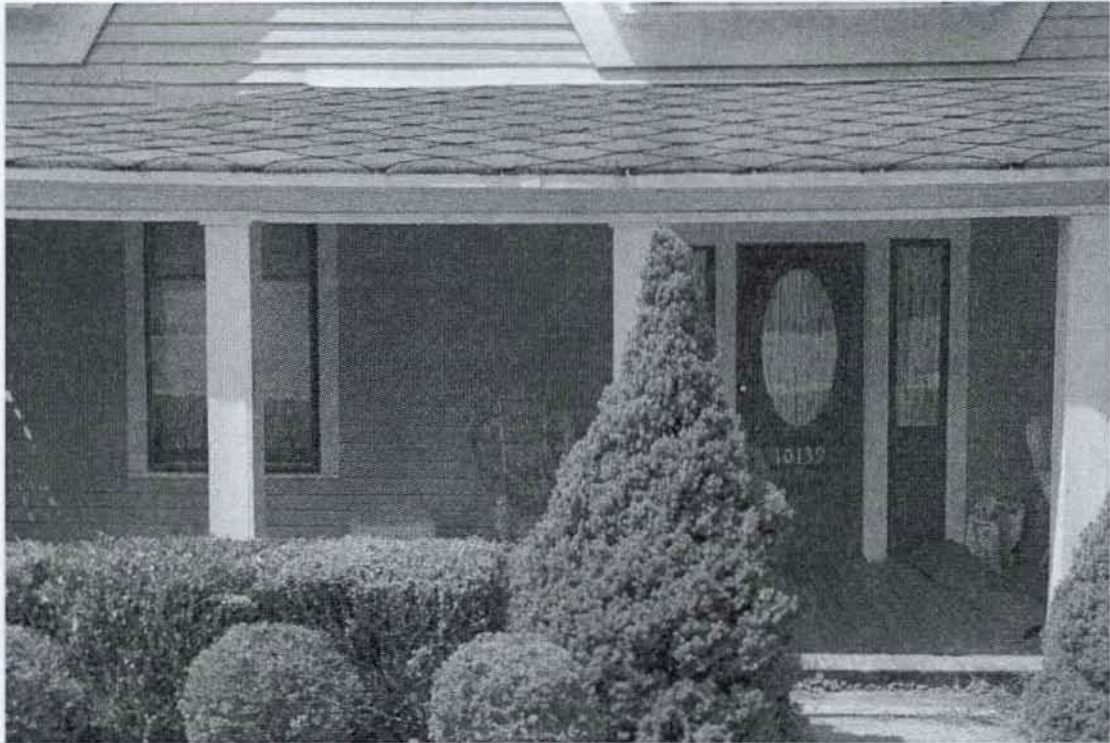
6. Exterior, south façade, detail, camera facing north 7. Photo #07
