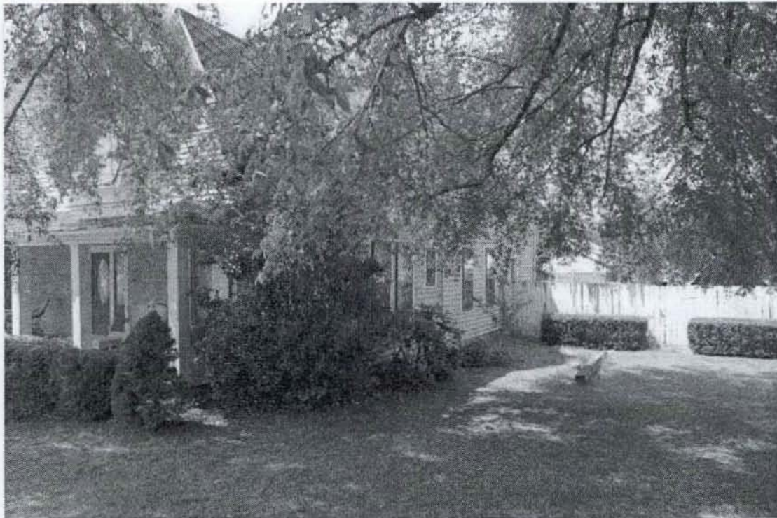
6. Exterior, south façade (left) and east elevation, camera facing northwest 7. Photo #05
