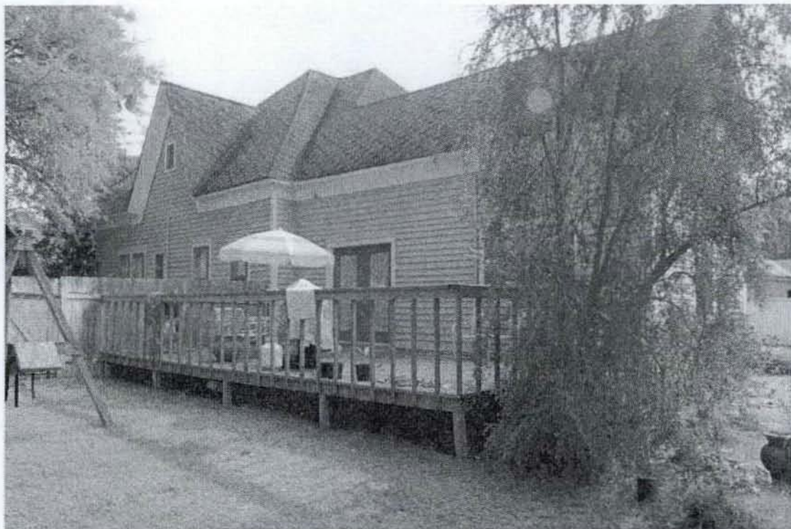
6. Exterior, east elevation, camera facing southwest 7. Photo #06
