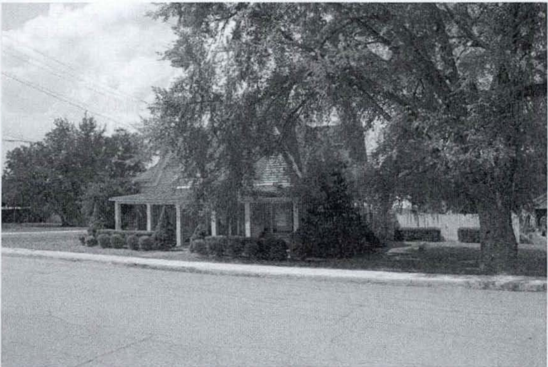
6. Exterior, south façade (left) and east elevation, camera facing northwest 7. Photo #04
