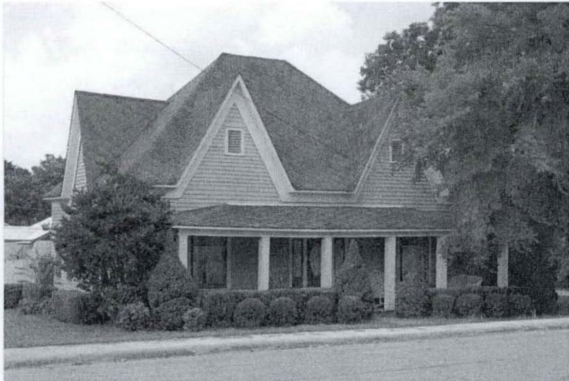
6. Exterior, south façade (right) and west elevation, camera facing northeast 7. Photo #01
