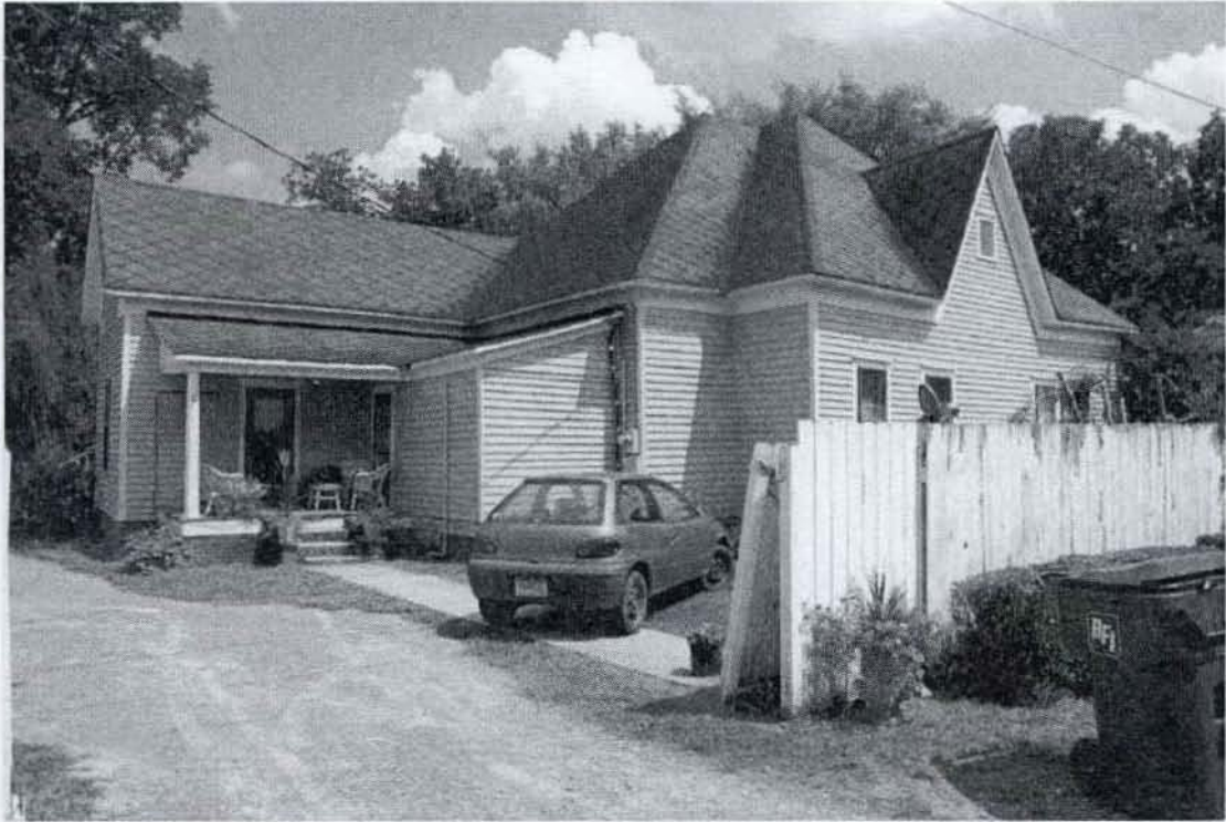
6. Exterior, north (left) and west elevations, camera facing southeast 7. Photo #03
