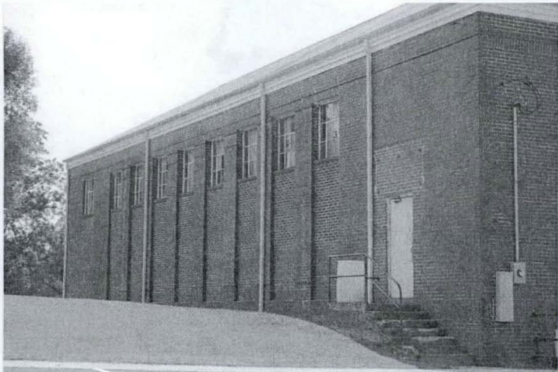
6. Exterior, east elevation, camera facing west 7. Photo #04
