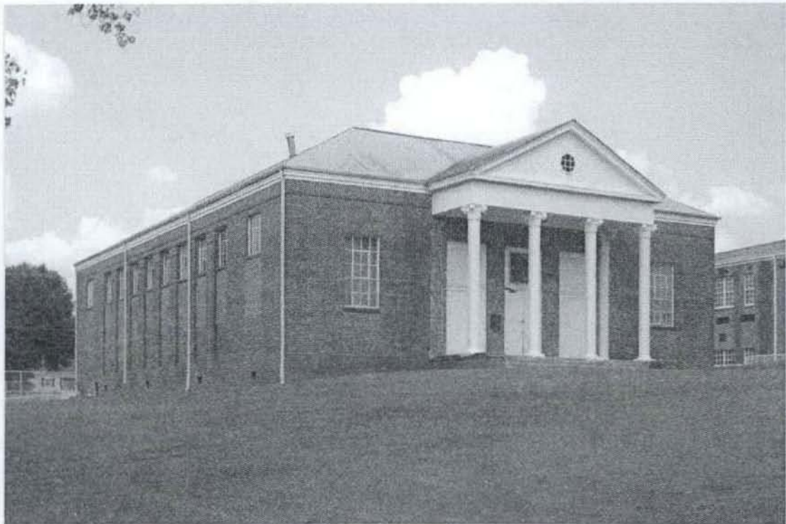
6. Exterior, west (left) and south (right) elevations, camera facing northeast 7. Photo #02
