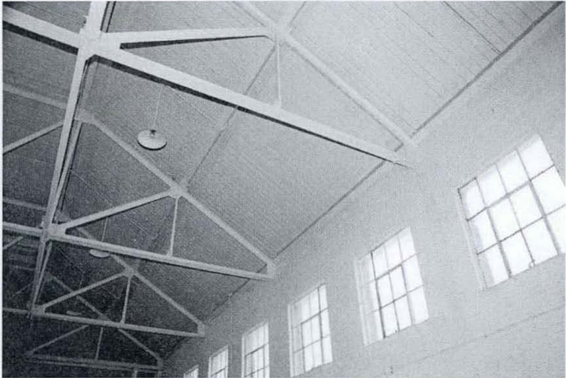
6. Interior, detail of roof trusses, camera facing northeast 7. Photo #13
