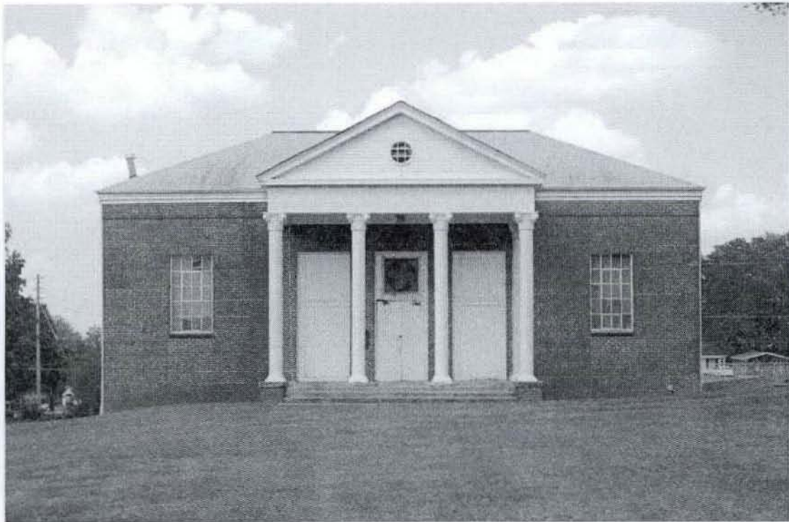
6. Exterior, East façade (right) and south elevation, camera facing northwest 7. Photo #01
