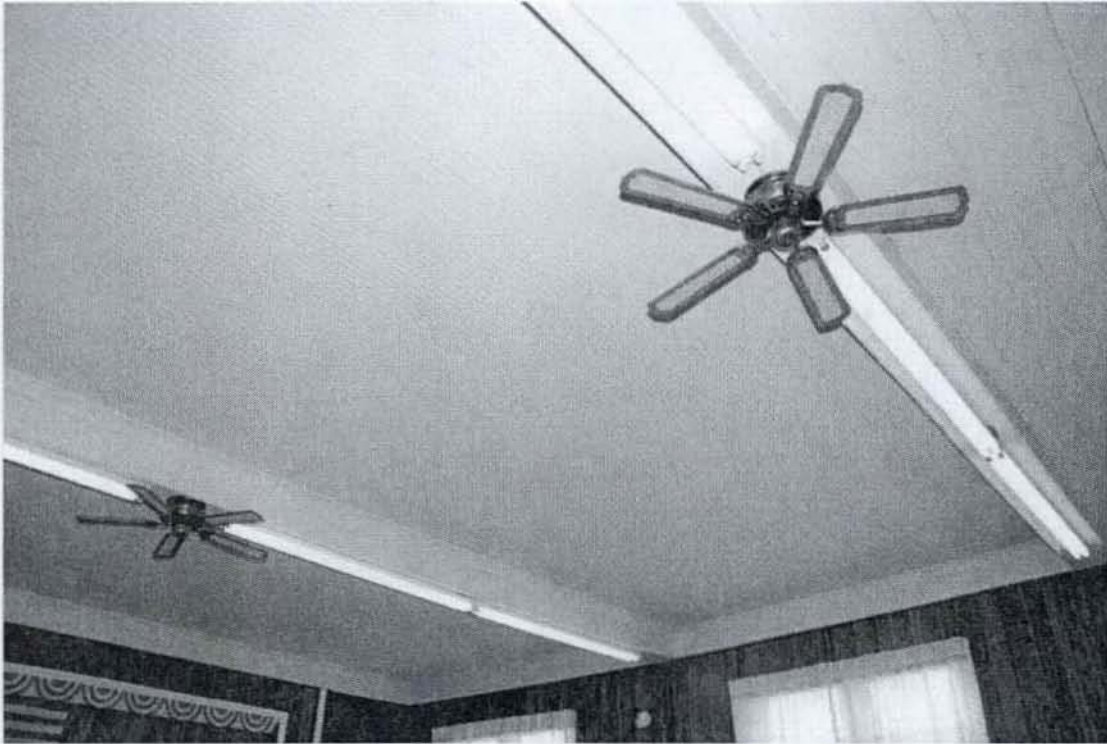
6. Interior, 1 st floor, Dining Room, detail of ceiling 7. Photo #07
