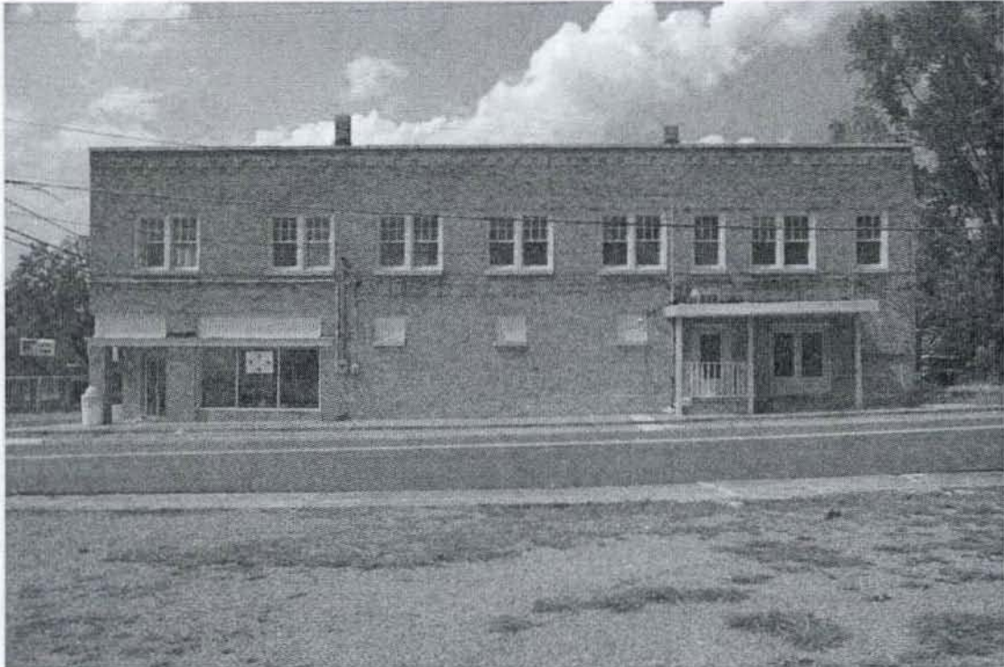
6. Exterior, south elevation, camera facing north 7. Photo #03
