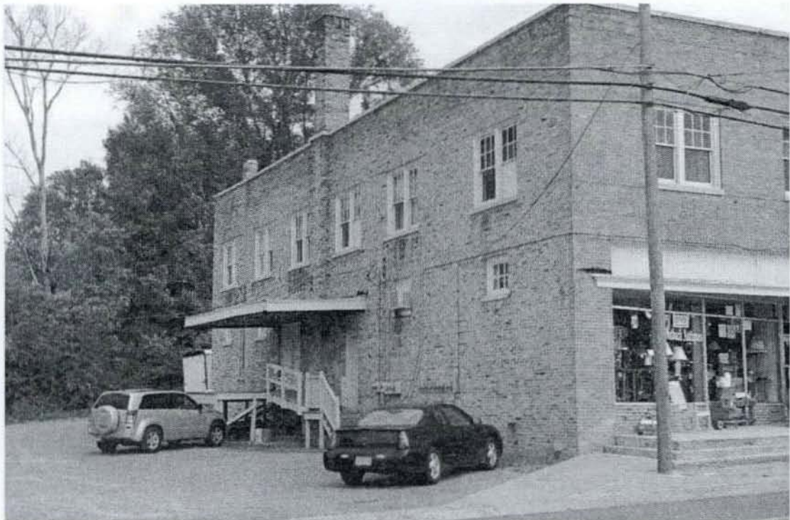
6. Exterior, north elevation, camera facing southeast 7. Photo #05
