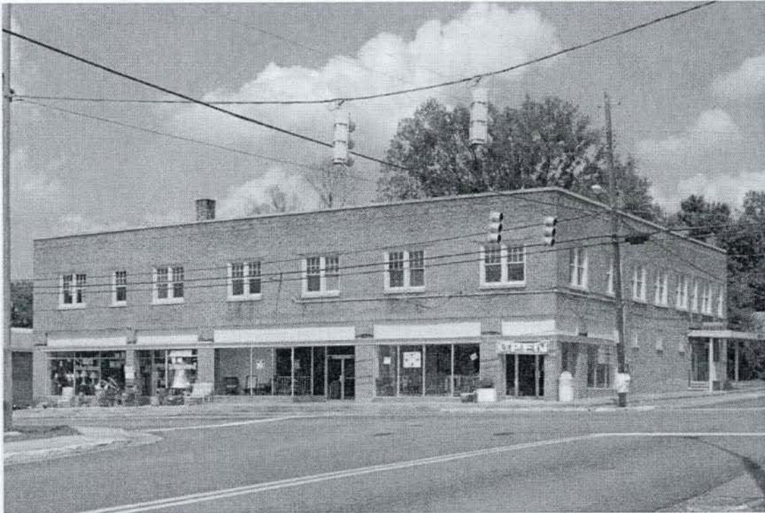
6. Exterior, West façade (left) and south elevation, camera facing northeast 7. Photo #01
