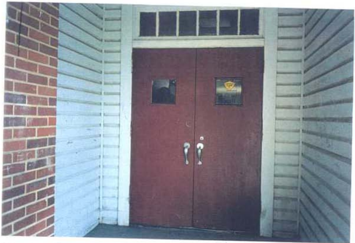
Back door northwest side of original building (LTS) 8-12-93
