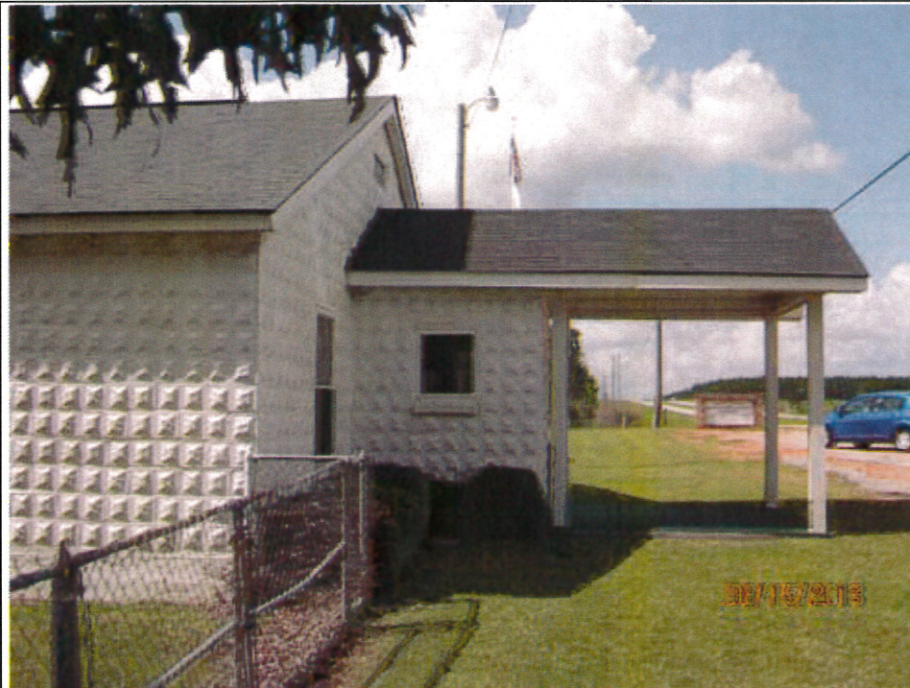
5. View looking north toward Halls Creek Missionary Baptist Church entrance.
