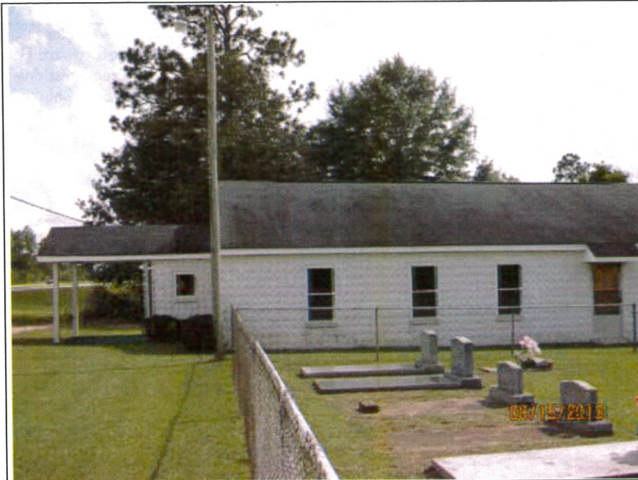
3. View looking southwest toward north facade Halls Creek Missionary Baptist Church.
