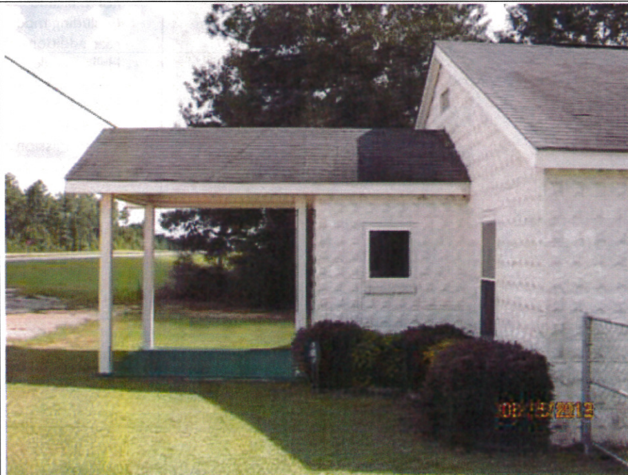
2. View looking south toward Halls Creek Missionary Baptist Church entrance.
