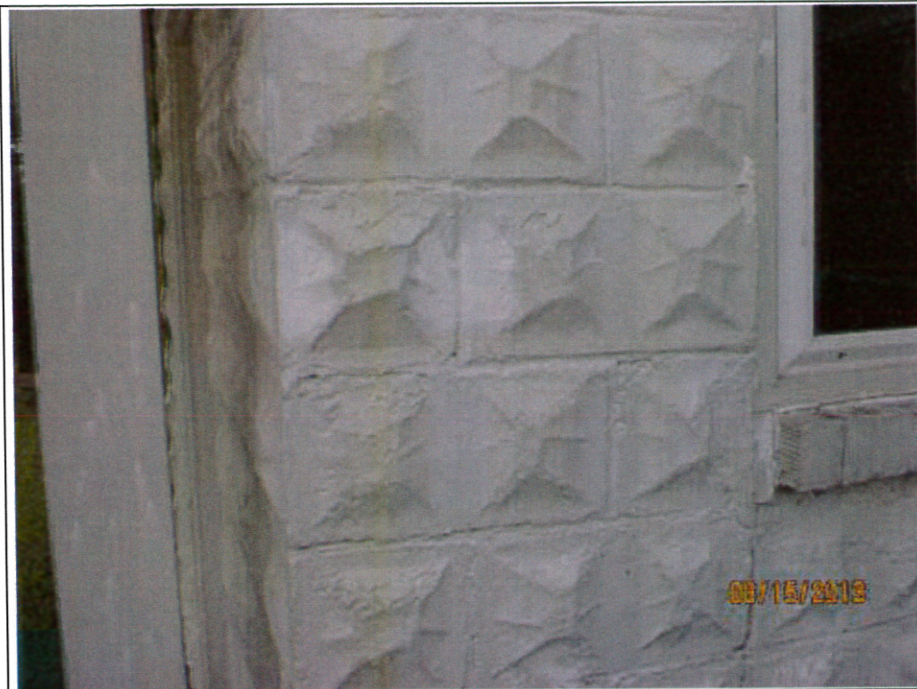
7. Detailed view of cast stone wall.
