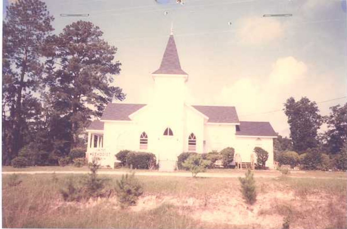
1926 & 1989 REMODELING AND EXPANSION -
